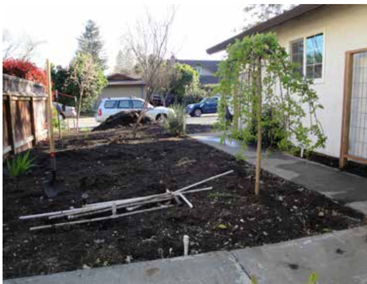
Modifying the existing irrigation system before getting started.
