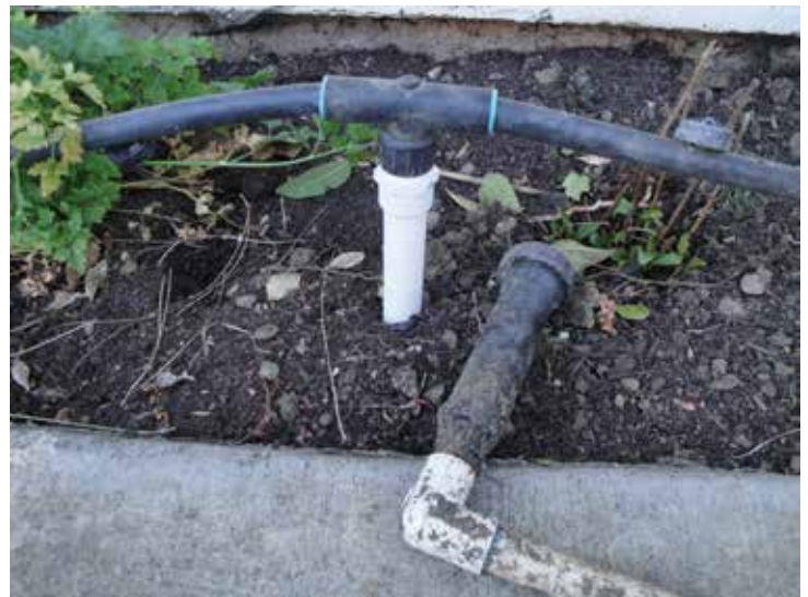
Plumbing new drip connections in place of overhead sprinklers.
